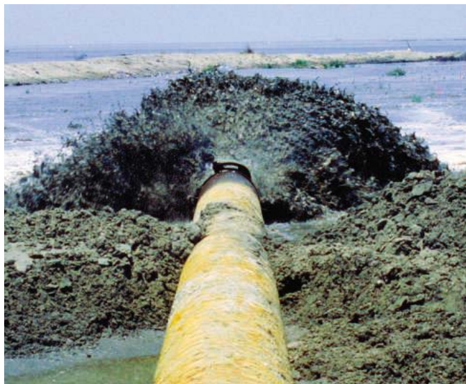
Gusher. Pumping sediment through pipelines can create tracts of wetlands, but ecologists doubt that the energy-intensive technique is sustainable.
